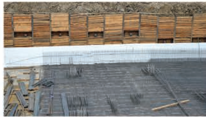
Shoring / Soil Stabilization
